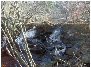
Pare Engineering of Foxboro, Ma. submitted a Phase II Inspection/Evaluation report to the Town that confirms the structural problems with the dam. They also have identified significant seepage beneath the actual dam structure. Pare has prepared cost estimates, accrued over twenty five years, of three options available to keep the dam in compliance with dam safety standards. Simple repair, though cheaper in the short term is cost prohibitive over time. (1)
