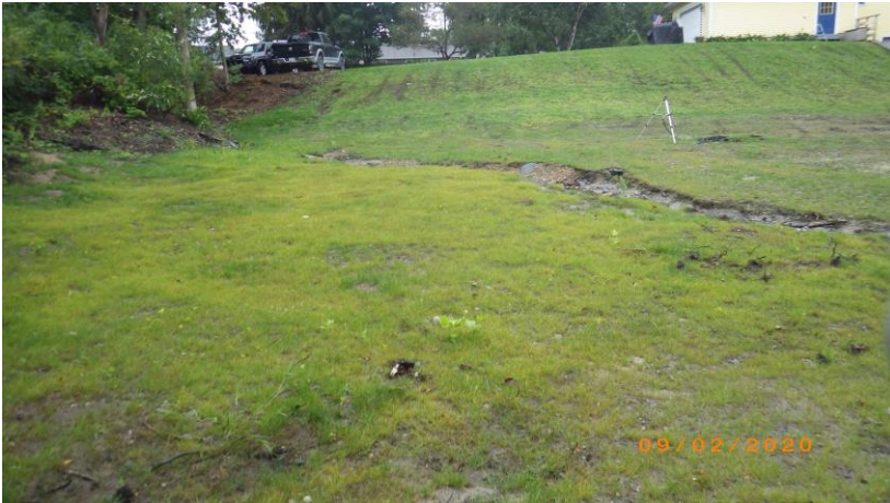
View north across cleared area showing channel developing from storm drain outlet
