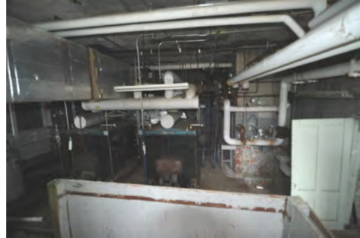
Mechanical room with asbestos laden piping and boilers.
