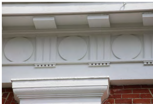
Top right: Main entry flanked by painted brick pilasters and surmounted by a transom window; door hood supported by console brackets. Left: Alternating triglyphs and metopes at the frieze. Right: Brick jack arches at windows, corner quoins and horizontal string course over windows.
