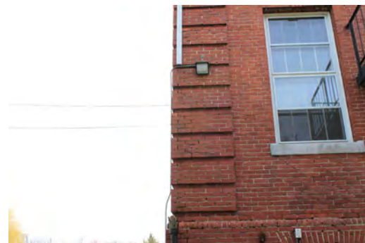
Broken downspout has caused severe deterioration to the mortar joints below
