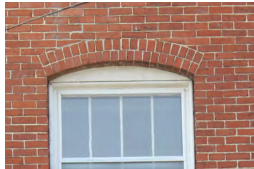
This facade is the only one which uses an arched lintel as opposed to a jack arch lintel.
