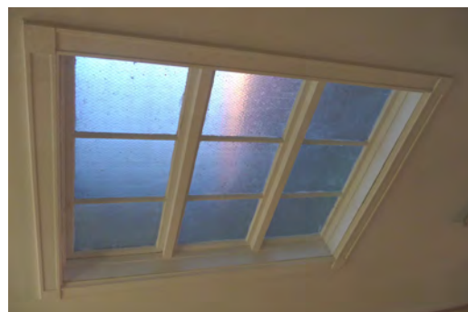
Laylight in second floor hallway with daylight coming through the roof skylight.
