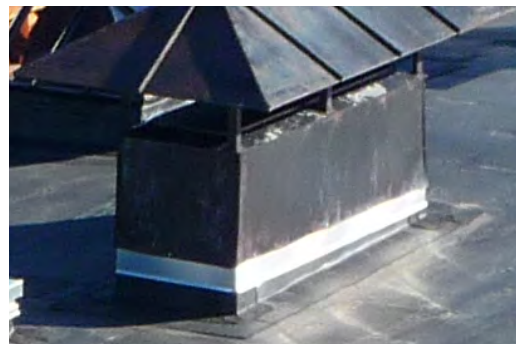
Flashing detail at ventilator.
