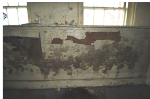
Mold on painted wainscot
