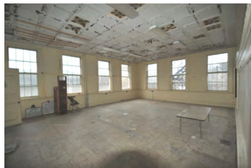
Classroom 3 on first floor, south east corner of building. This room has remnants of a tin ceiling, with acoustic panels glued to it.
