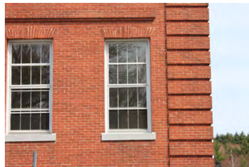
Top right: Main entry flanked by painted brick pilasters and surmounted by a transom window; door hood supported by console brackets. Left: Alternating triglyphs and metopes at the frieze. Right: Brick jack arches at windows, corner quoins and horizontal string course over windows.
