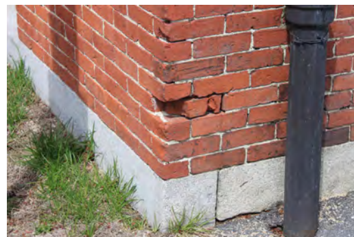
Dislodged bricks at the northeast corner.
