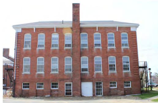
East elevation - note staining beneath windows
