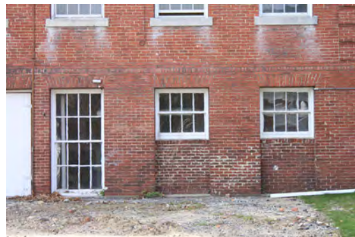
Rear elevation. Brick efflorescence, evidence of water infiltration, under the window lintels and poorly executed repointing at the basement level.
