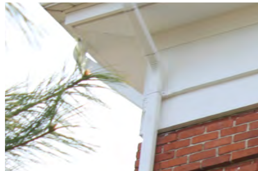
Two corrugated aluminum downspouts joining at northeast corner.
