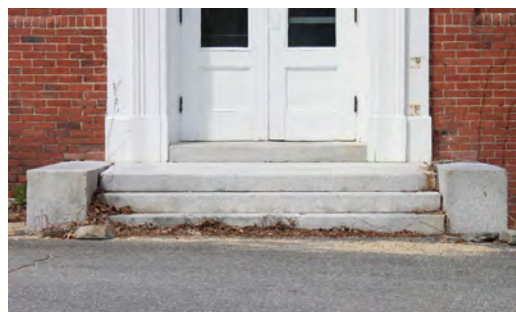
Shifted, separated granite steps at the north elevation.
