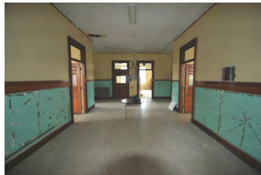
Second floor hall with damaged wainscot paneling.
