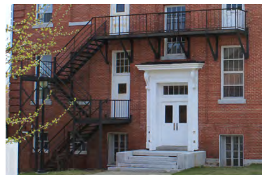
Steel fire escape and brackets are deteriorating. Three original window openings were converted to doors for access.
