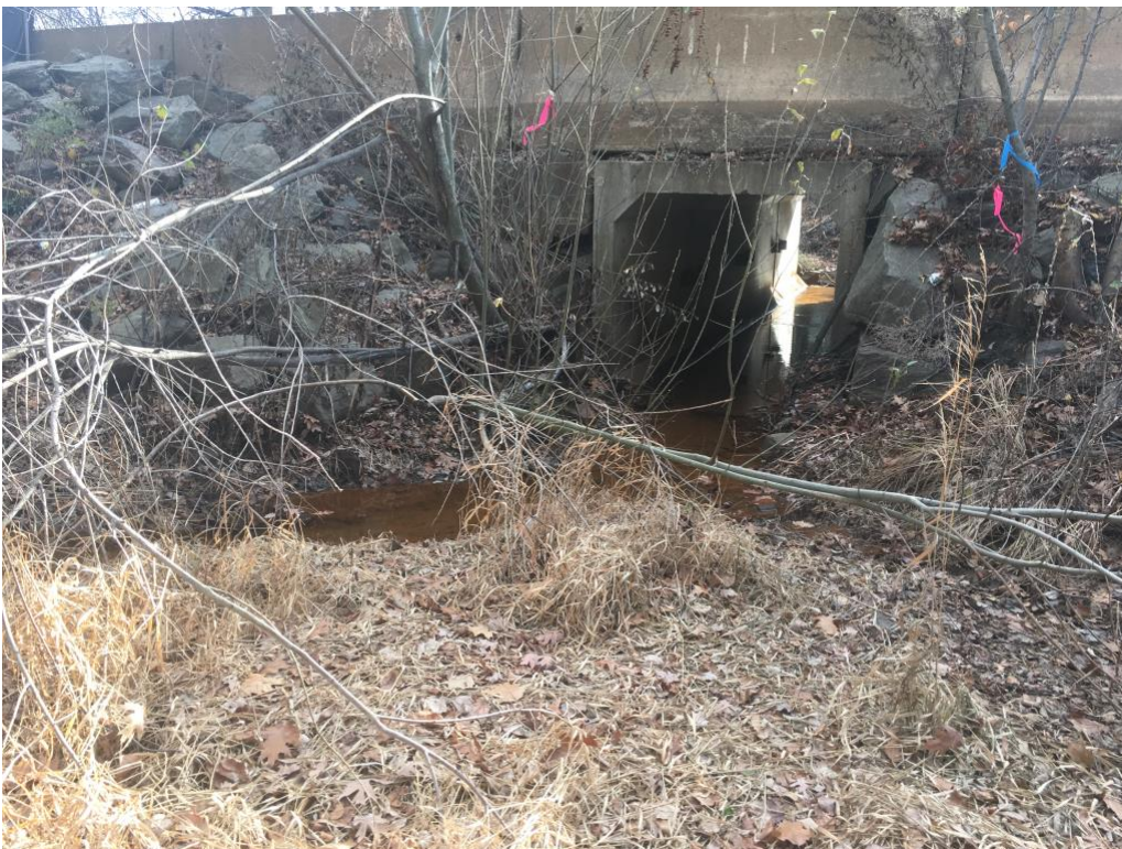
Photo 3: Upgradient of existing stream crossing on McGovern Blvd, 11/19/2020
