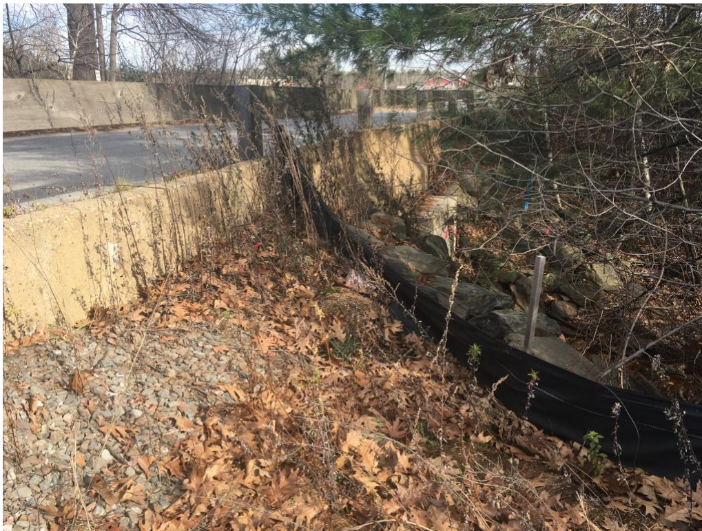
Photo 1: Existing stream crossing slope on McGovern Blvd, 11/19/2020
