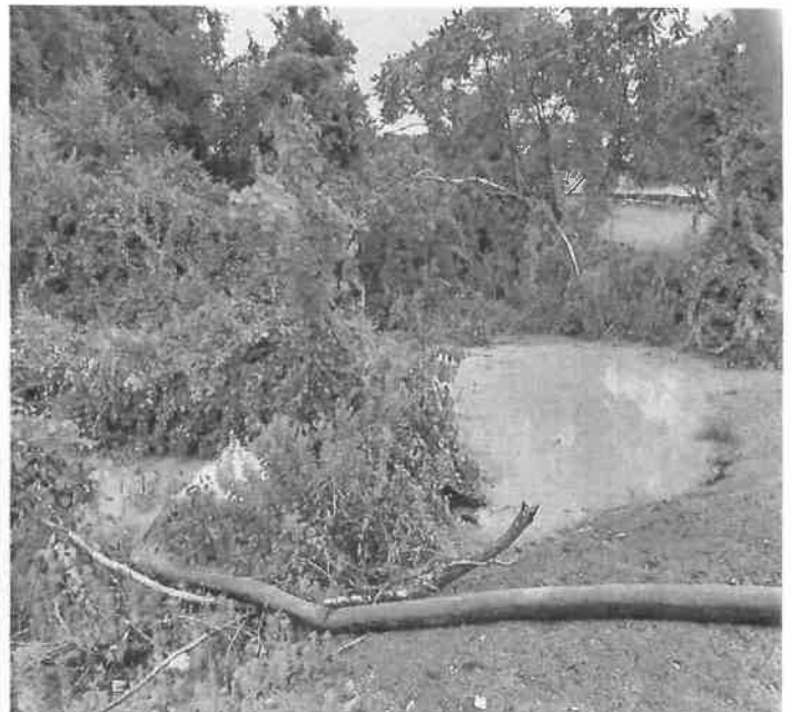
#6 Turbidity & Silt Discharge into Buffer Zone & Wetland
