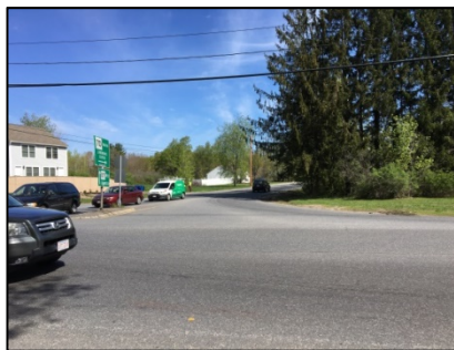
Image 7: Wide turn radii for heavy vehicles leads to high turning speeds for personal vehicles
