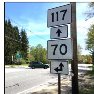
Image 4: Guide signage heights below 7-foot minimum set by MUTCD standards
