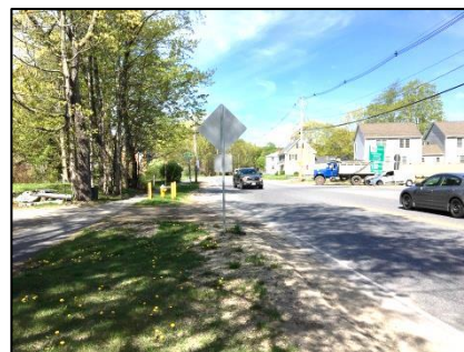
Image 2: Variable width grass buffer with lack of vertical separation for sidewalk along southerly side of Main Street
