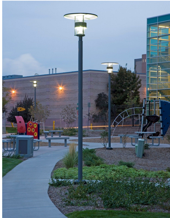
Pedestrian area lighting using 12-foot-tall poles
