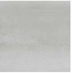
GROUT CLEANED CONCRETE
